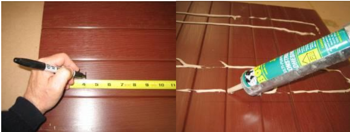
Images 5&6: Mark backer location & apply adhesive
