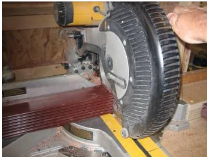
Image 3: Trimming the 3" T&G to the correct height
