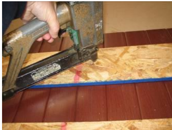
Image 9: Staple the backing board to the T&G pieces
