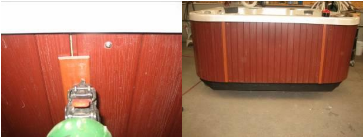
Images 19&20: Staple trim into position (covering gap between side panels & corner section). Note: trim strips are shown in a different color to highlight their location.
