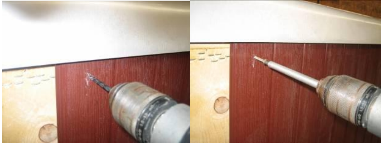
Image 15&16: Pre-drilling the panel & screwing it into position
